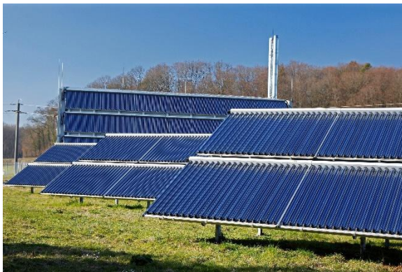
Figure 5: Ground mounted evacuated tube collectors in Büdingen, Germany (Solites)
